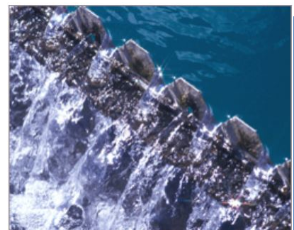
Weymouth Treatment Plant
