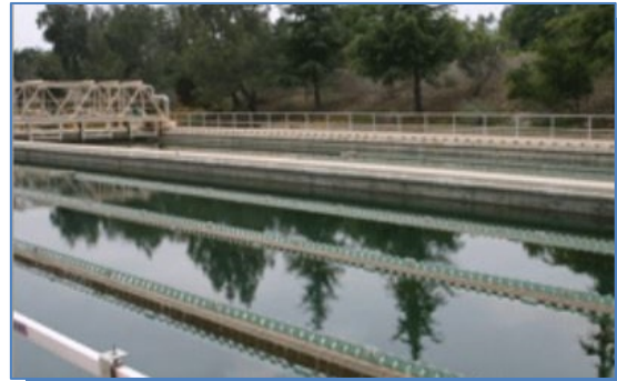
Miramar Treatment Plant
